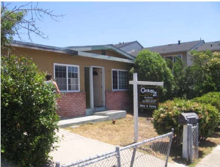
West Facing Elevation (City lights and ocean / bay views from kitchen / dining area not shown.)
